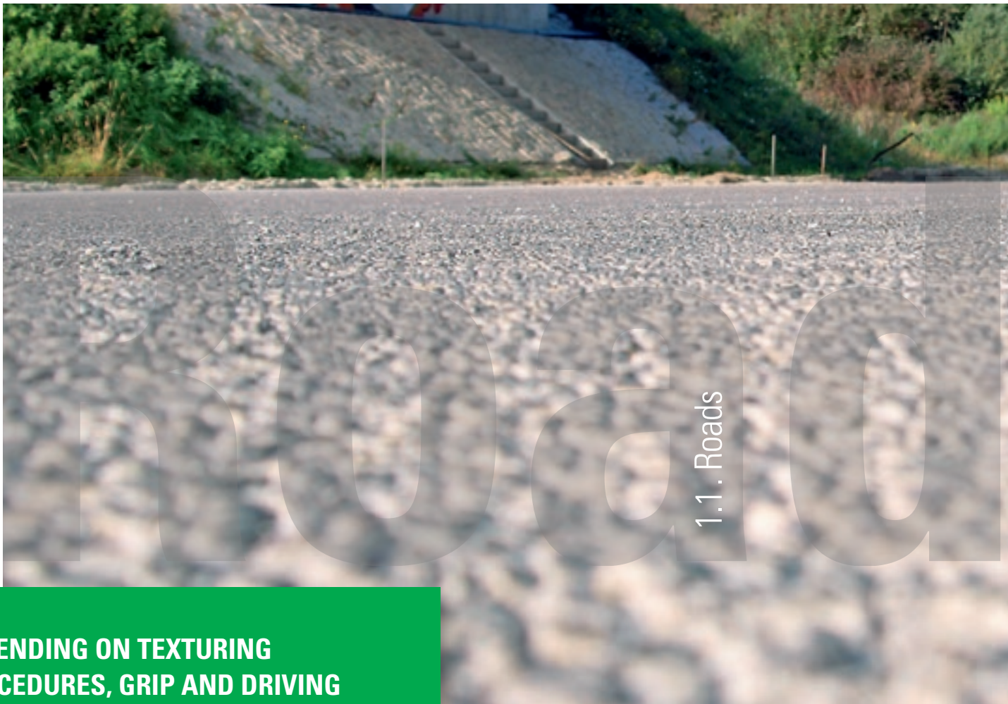
Detailed view of exposed aggregate concrete surface ↓
