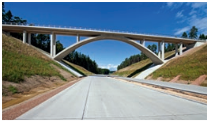
↑ Road surface and arched bridge, B15 Regensburg to Landshut
