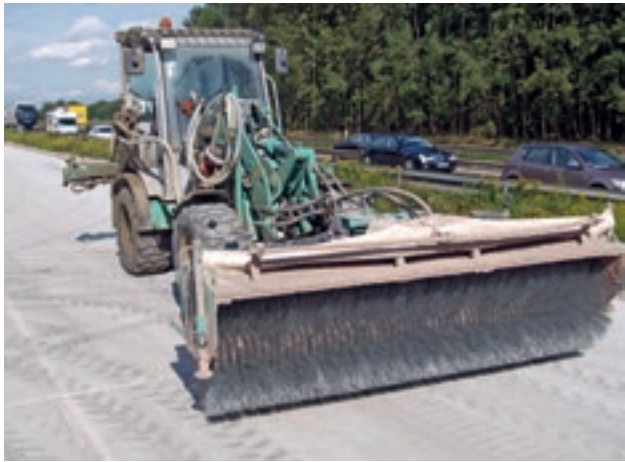
Manufacture of the exposed aggregate concrete surface by brushing ↑
