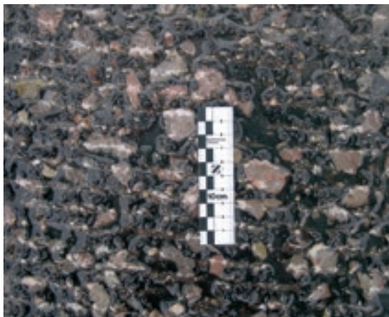
Detail of a milled, wet-cleaned asphalt surface →
