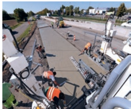
↑ Concrete construction with the slipform finisher, B47 Bensheim ↓
