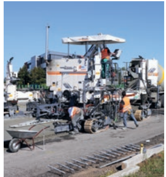
↑ Concrete construction with the slipform finisher, B47 Bensheim ↓
