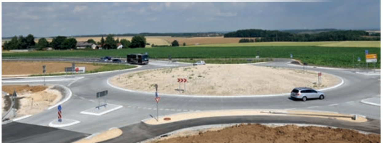
↑ Concrete roundabout, Ulm-Langenau, BAB A8 – AS Ulm-Ost
