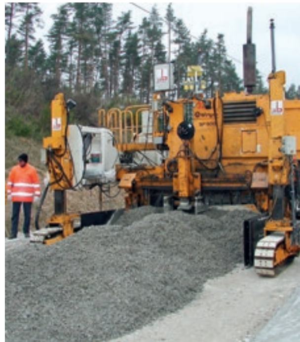
↑ Construction of the HBB with a slipform finisher
